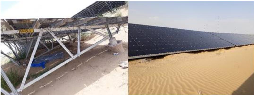
*Figure 2: Soil Erosion and Accumulation due to high wind*
