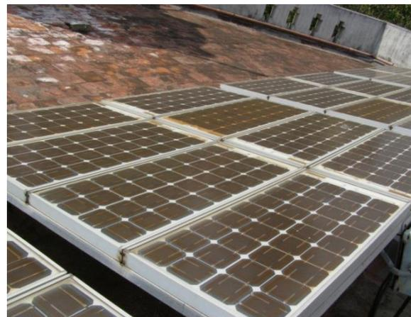
*Figure 4: PV Module indicating Discoloration*
