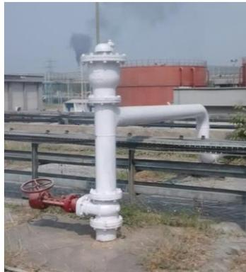
**Figure 3. Hot water blow down tapping from Air Release Valve (ARV)**
