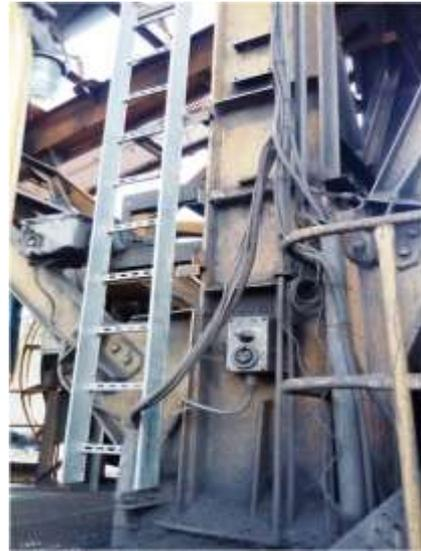
Fig.7:- New Cable trays laid
