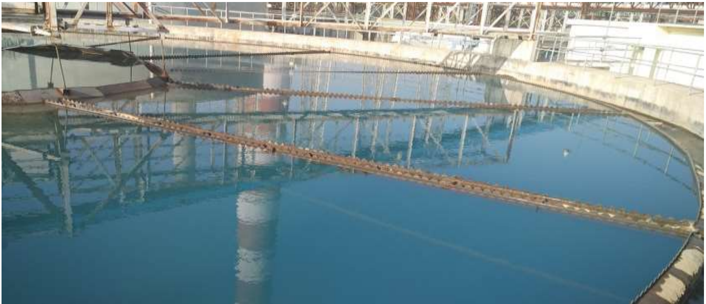
Improvement in CW Clarifier water quality after polyDADMAC dosing
