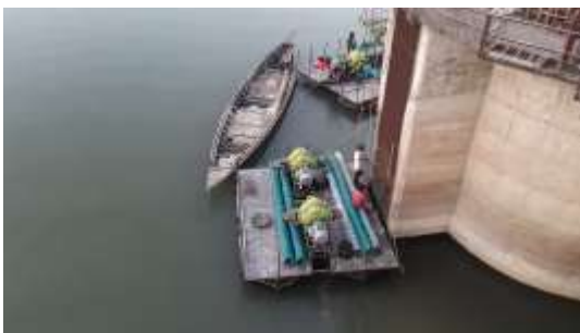
Fig-1 (Barge Pump under erection)
