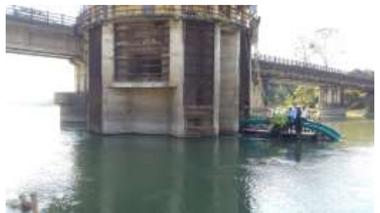
Fig-2 (Barge Pump under erection)
