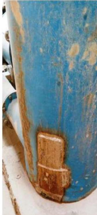
Repaired by Patch welding
