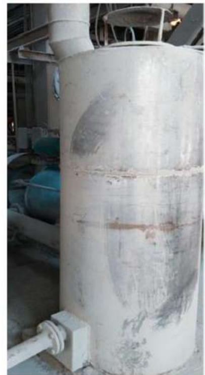
Stainless steel silencer Fabricated at site
