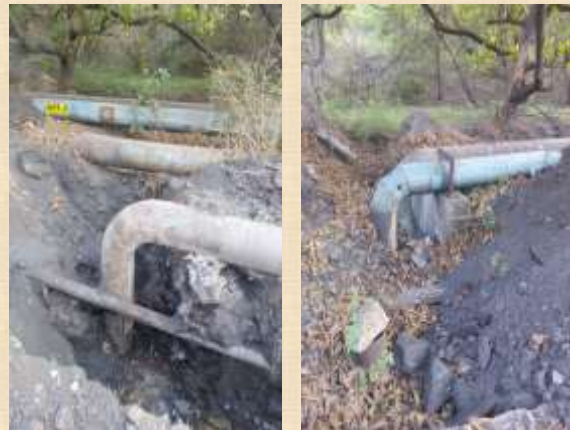
Pipes under earth
