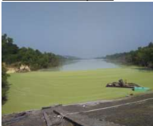
Clean water after settling of ash
