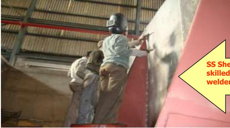
**SS Sheets are fitted in the wagon by the skilled fitter with the help of certified welders**
