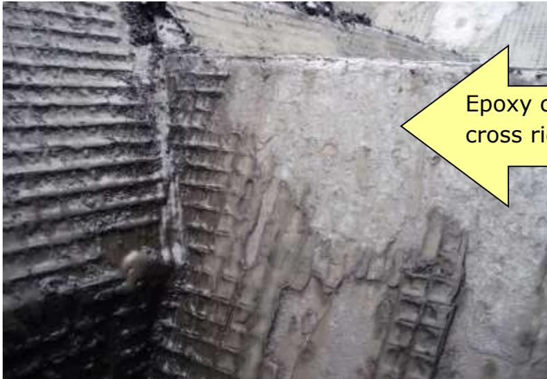
Epoxy coating peeled off from cross ridges
