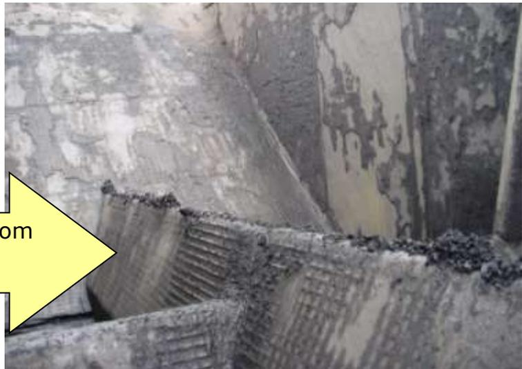
Epoxy coating peeled off from longitudinal ridges
