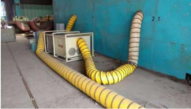
Photo-2 Air conditioning system supplying fresh cold air to enclosure
