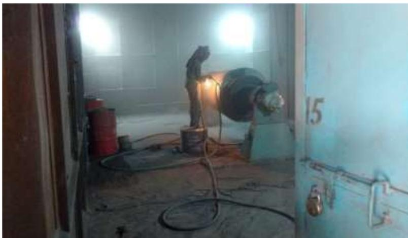
Photo-4 Actual Site Photograph during Alumina blasting with improvised system
