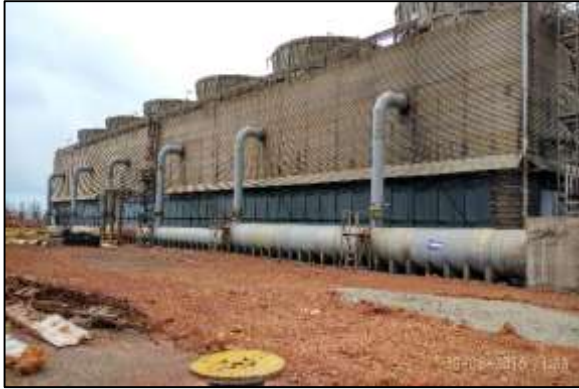
Figure – 4: Hot water manifold before and after modification.
