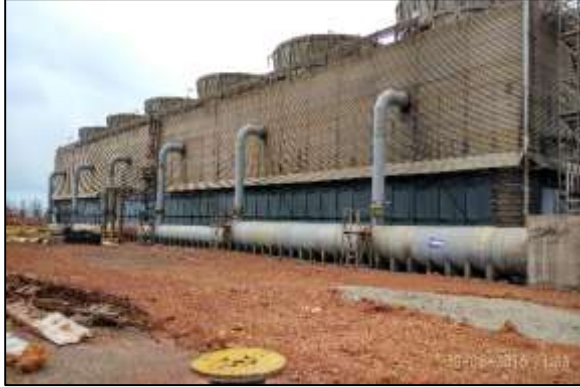
Figure – 1: Hot water manifold before modification.
