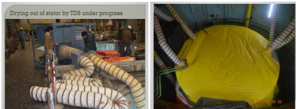
Figure-1: Dry out of stator through hot air blower
