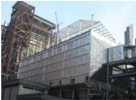
Renovation of ESPs of Stage I & II units are in progress with a target to lower the SPM values better than the statutory norms. After R&M, guaranteed SPM value in unit 1 to 6 shall be 75 mg / NM<sup>3</sup> and Unit-7 & 8, SPM shall be 68 mg/NM<sup>3</sup>. The contract for this renovation job has been awarded to M/S BHEL and the work will be completed by Dec 2017.
