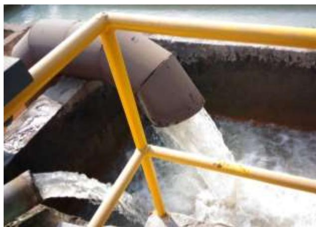
Fig. 1 Use of standby clariflocculator for recycling waste water.
