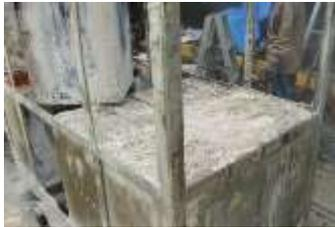
In the first step the catalyst elements (boxes) have been removed from the modules and mechanically cleaned. This is very important as between the elements heavy dust deposit occurs and to ensure full performance with low pressure drop this plugging shall be removed.
