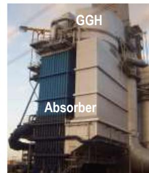
**Fig.4-4 GGH on the absorber**
